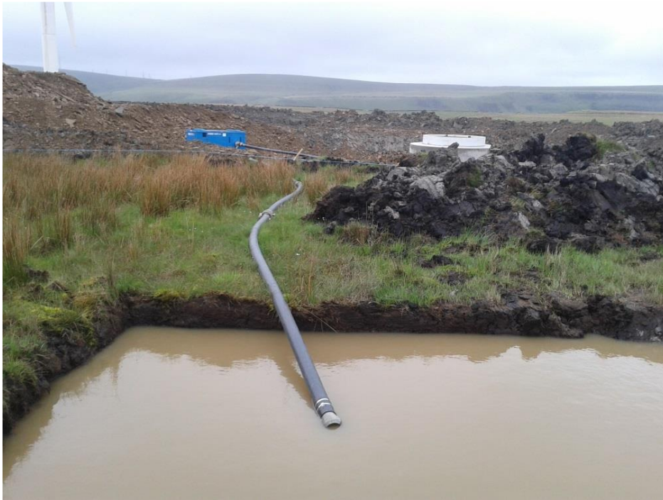
Plate 6: Typical 'Siltbuster' and settlement lagoon
