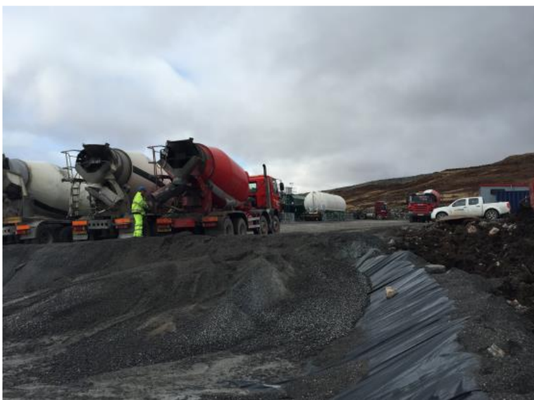
Plate 10: Typical concrete wash-out facility
