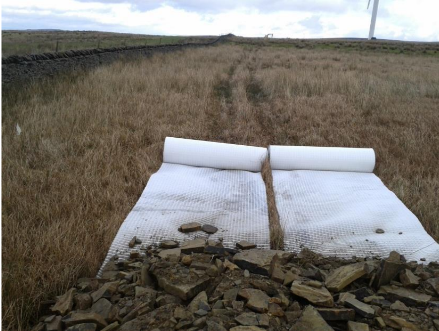
Plate 13: Semi-permeable geotextile layer
